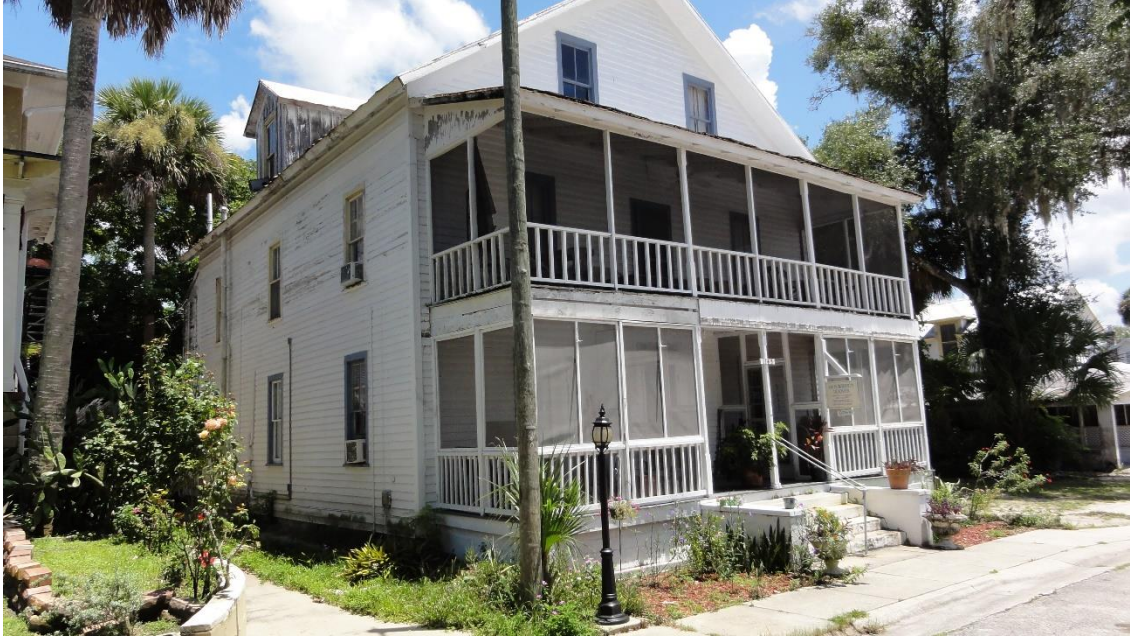
(above) Brigham Hall (apartment building); (below) Caesar Forman Healing Center.
