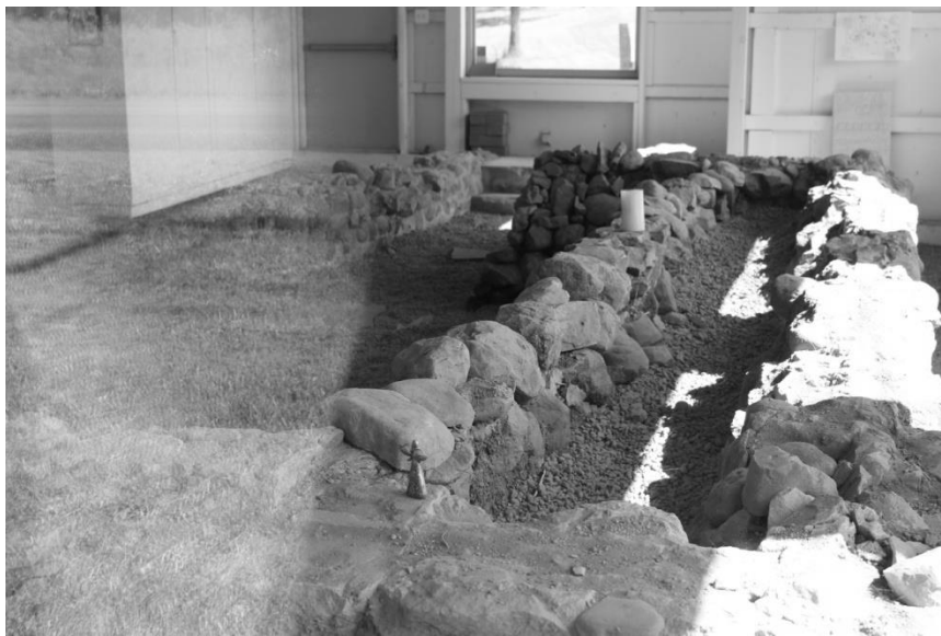
[Illustration 4: Original foundation of the Fox Cottage; photo taken June 2015.]
